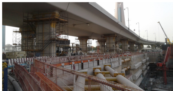
Online monitoring of existing bridge, deep excavation and new structure construction, with geotechnical and geodetic instruments
