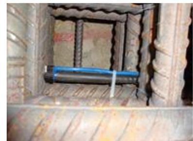
Route the sensor cable along the reinforce bar to the junction box, tying it at every 1 m with nylon cable ties. Do not use soft iron ties on cable as it can cut the cable.
