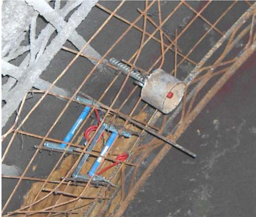
Photo 1 A pair of Encardio-rite model EDS-30V shotcrete strain gages and convergence bolt of an optical target installed before shotcreting of an NATM tunnel.
