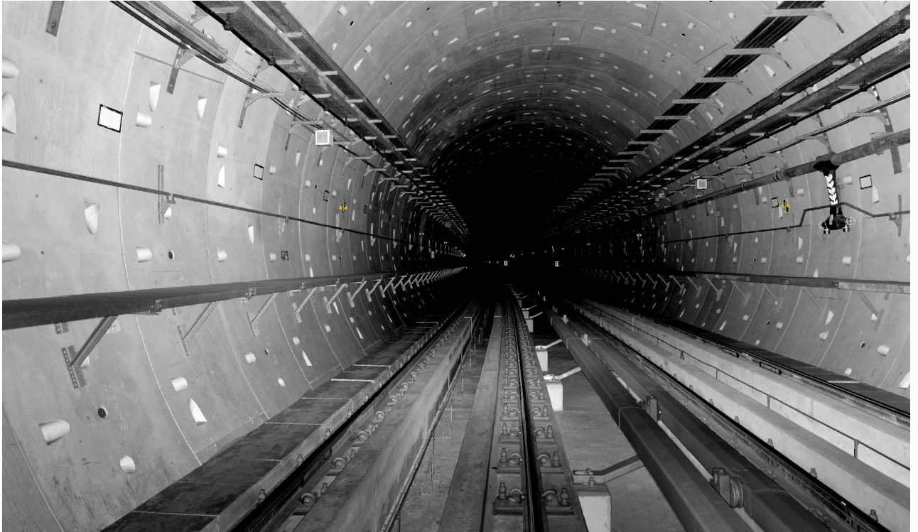
FIGURE 9 LASER SCANNING OF A TUNNEL
