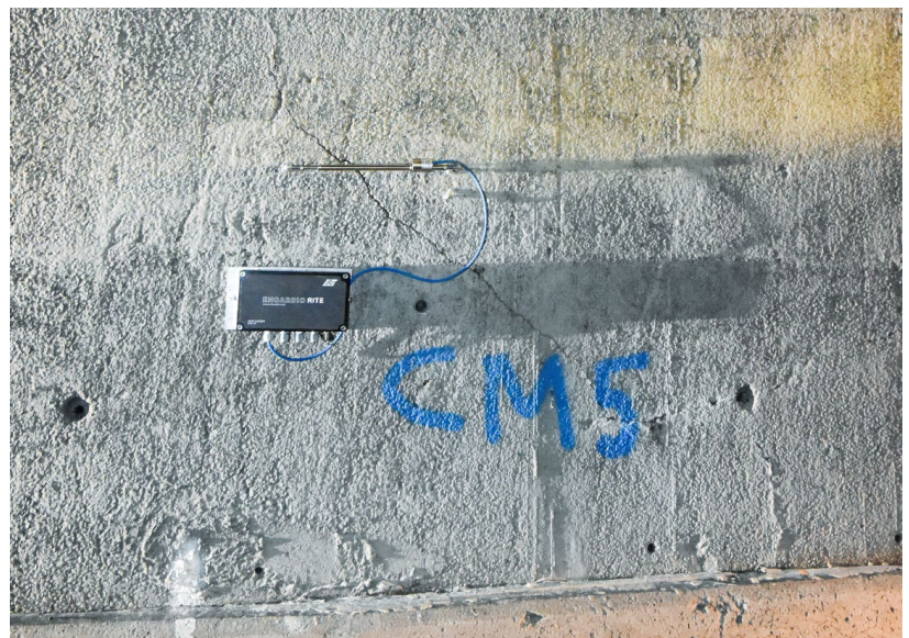
Crack meters installed across existing cracks
