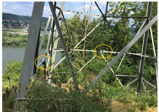
Tilt meters installed on the tower
