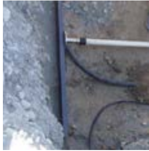
SOIL EXTENSOMETER BEING INSTALLED IN AN EARTH AND ROCKFILL DAM
