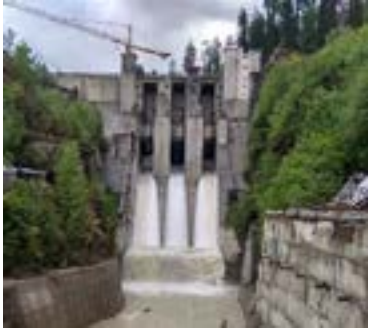
Parbati Concrete Dam, India
