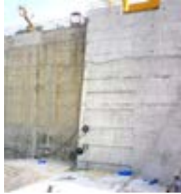
Sensors being installed at Middle Marsyangdi Dam, Nepal
