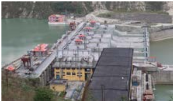
Teesta Concrete Gravity Dam, India
