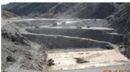
Work in progress at Salma Dam, Afghanistan
