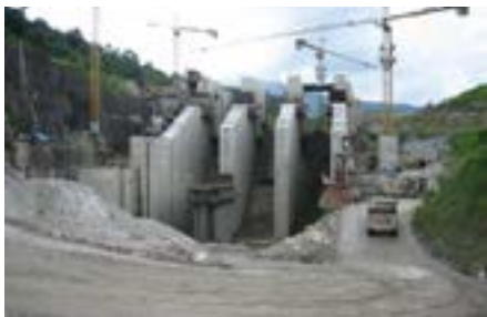
Work in progress at Middle Marsyangdi Dam, Nepal
