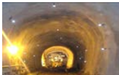
Prism targets in HRT at Dagachhu HEP, Bhutan
