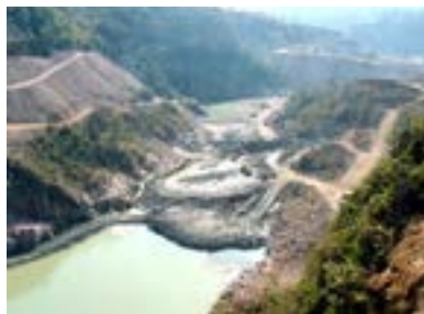
Work in progress at Middle Marsyangdi Dam, Nepal
