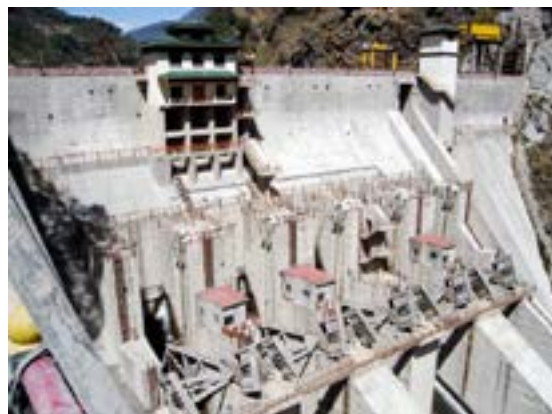
Tala concrete gravity dam, Bhutan
