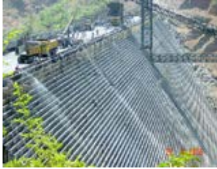
Ghatgar RCC Dam, India
