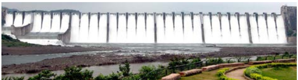
Sardar Sarovar Concrete Gravity Dam, India
