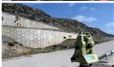
Automatic surveying system (ATS)
