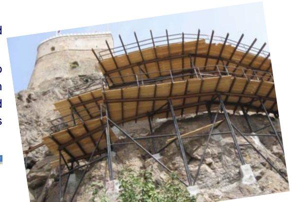
SCAFFOLDING FOR INSTRUMENTATION & PRESSURE GROUTING
