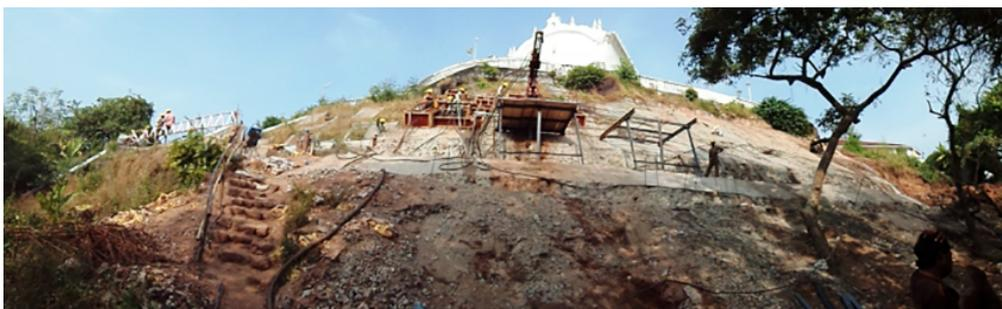
In-place inclinometers and piezometers installed for online slope monitoring at Cabo Fort, India
