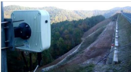
Gateway installed for wireless monitoring
