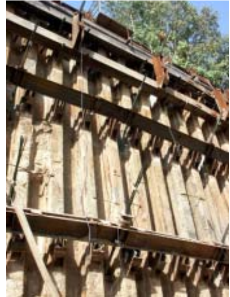
Figure-3 Sheet pile wall
