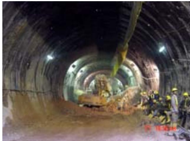
Figure-5: NATM tunnelling
