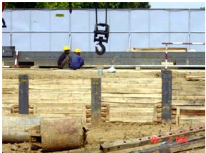
Figure-2 Soldier pile wall
