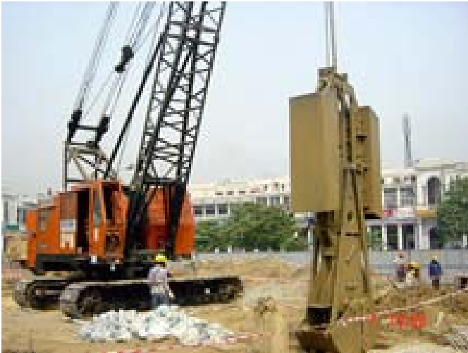
Figure 1: Trenching work for D-wall under progress
